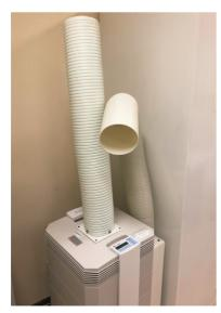
Figure 6 Portable HEPA filter unit.
